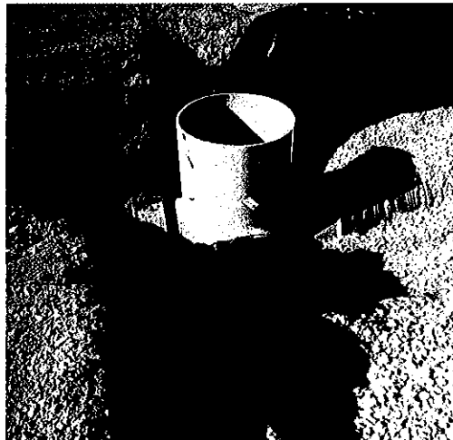
Nyloplast drain basins connect to perforated pipes in the subsurface stormwater retention system. Two workers can place the lightweight HDPE components, eliminating the need for cranes.
